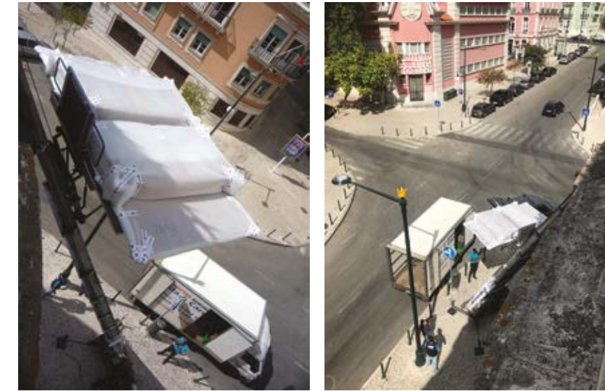
Desk modules (Cat. 26) being removed through a window of Casa-Museu Medeiros e Almeida on a platform lift.
