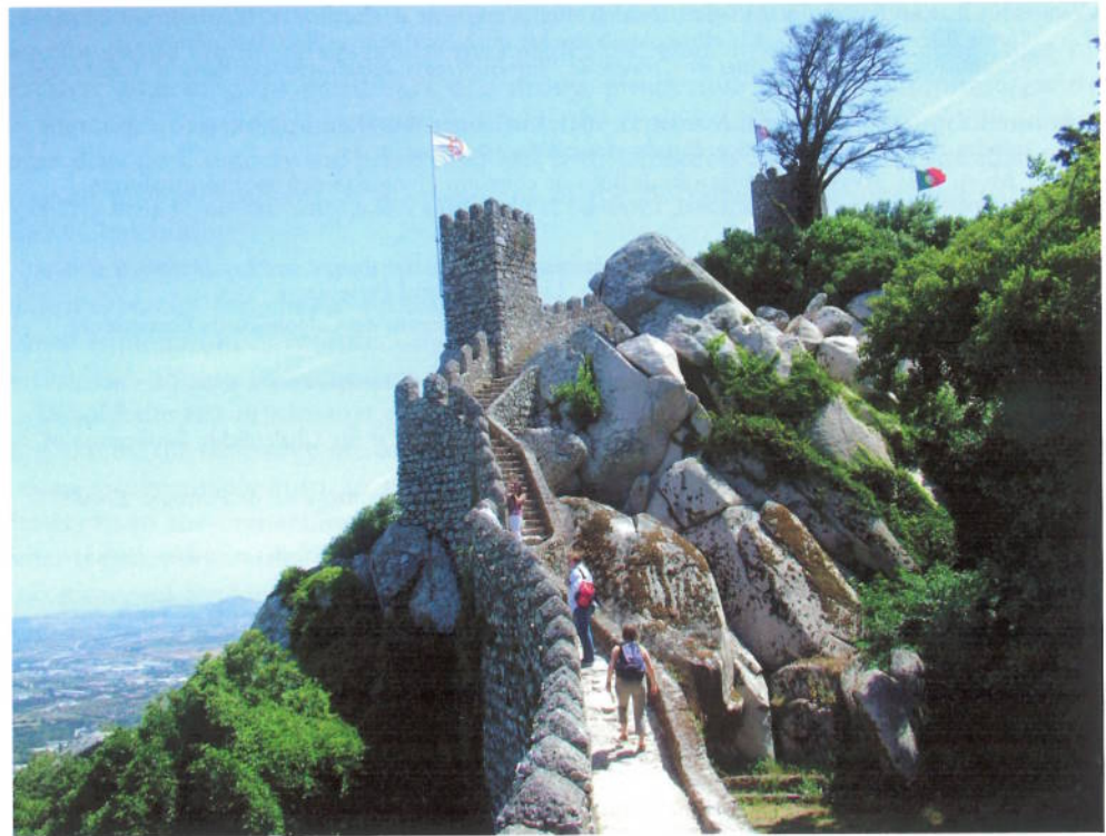
ILLUS. 22 Sintra, Castelo dos Mouros: general view of the rebuilt walls
