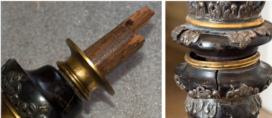
[fig. 42] Broken pieces on post A and post D. © Archeofactu
